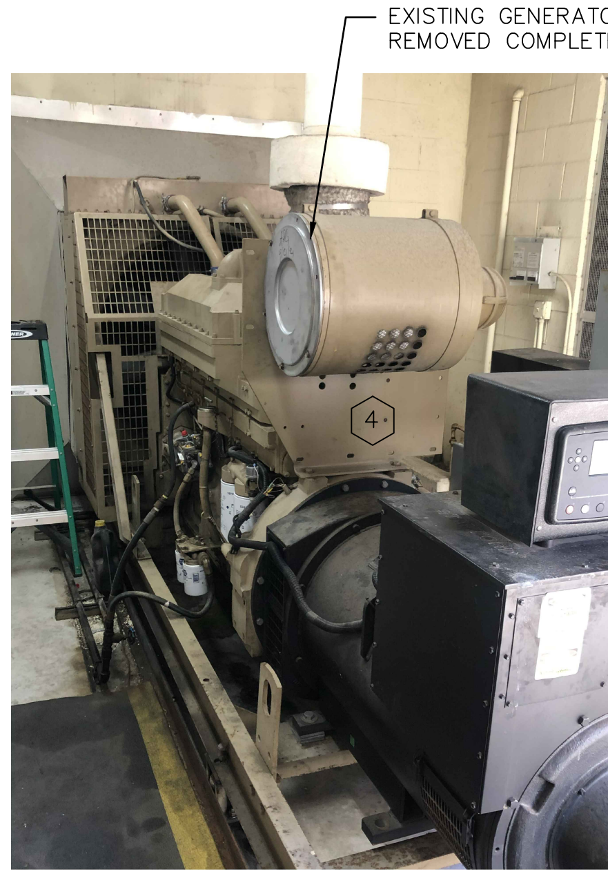
GENERATOR BUILDING PHOTO 3
