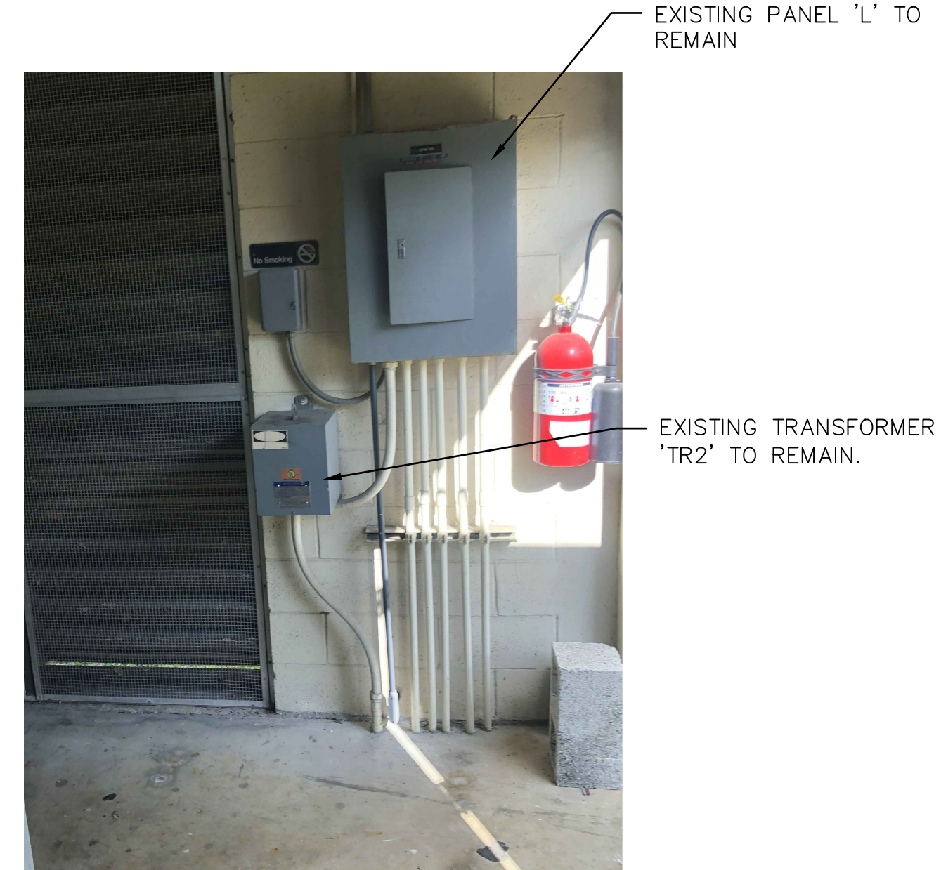
GENERATOR BUILDING PHOTO 2
