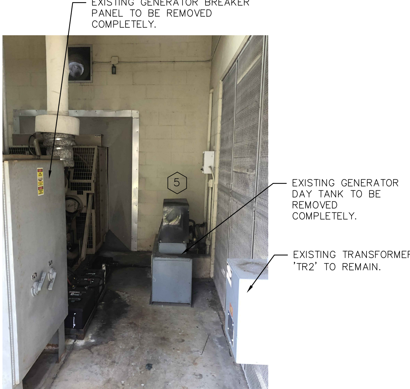
GENERATOR BUILDING PHOTO 4
